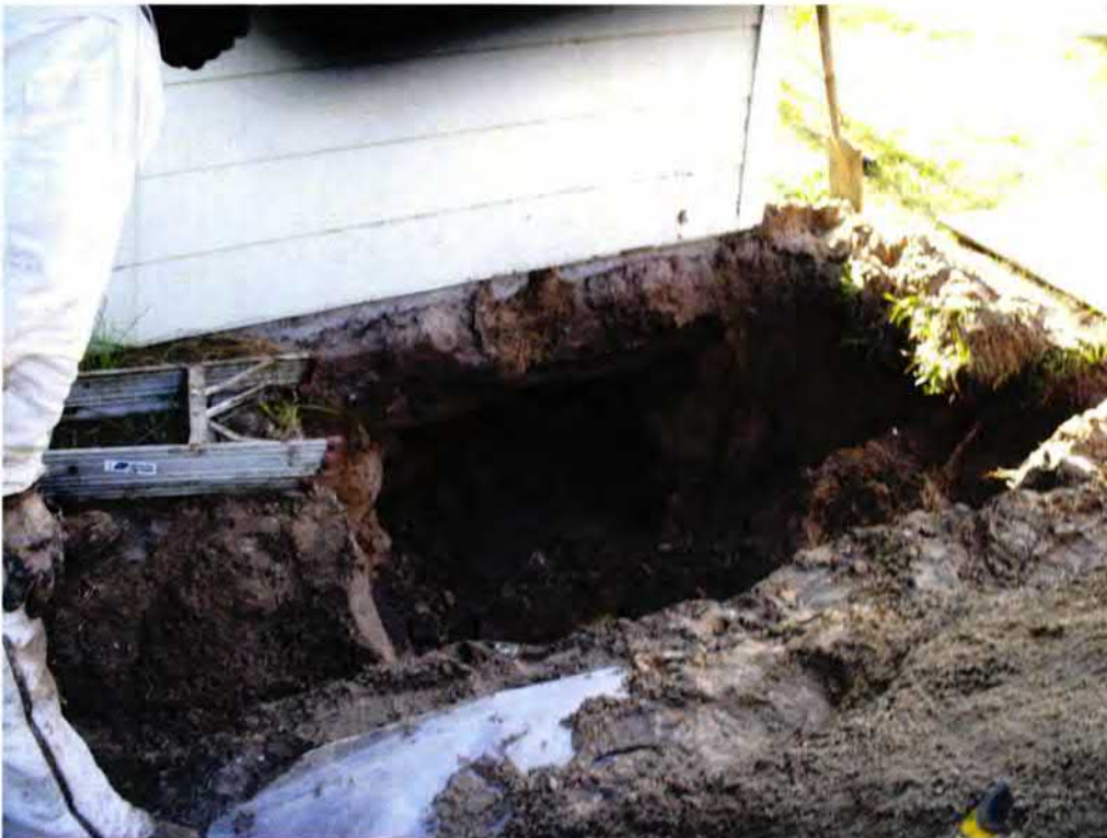
Picture 2: UST 418Elderberry removal in progress.
